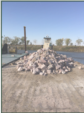
Rip rap as it is loaded on the barge.
