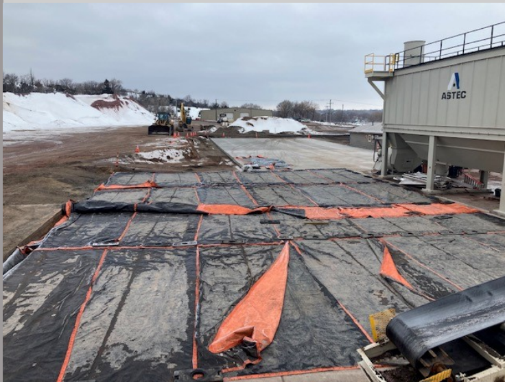
Rap system foundations.
