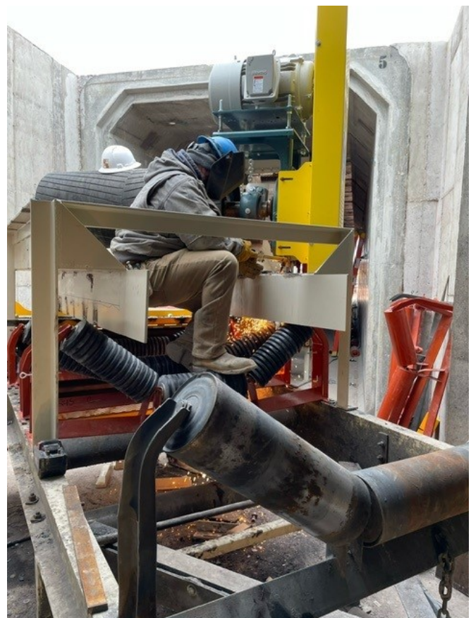
Carson Weideman at DRW modifying a head pulley.
