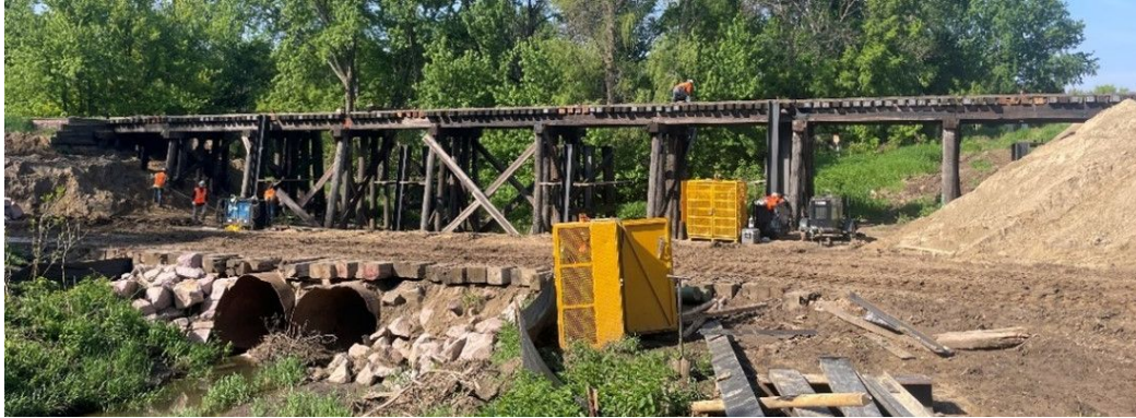
Timber bridge T-638 before replacement.
