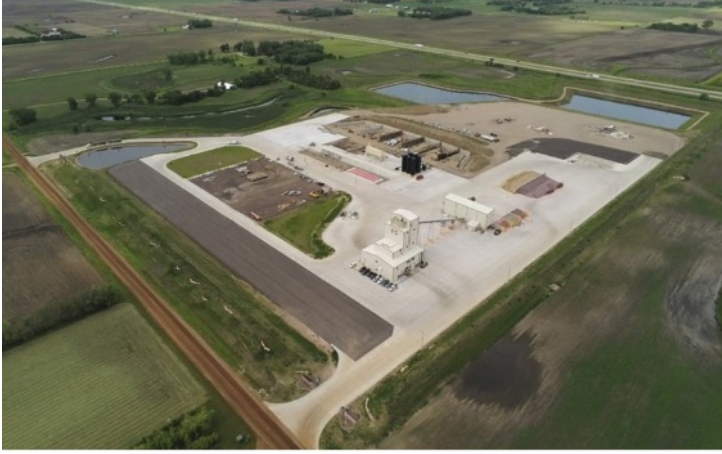
Nine Mile Park - a challenging project with beautiful results
