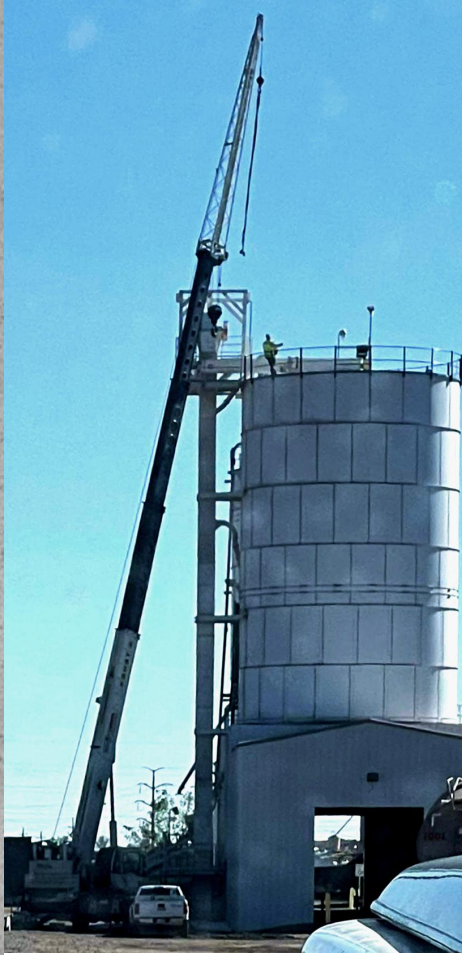
The crane installing the trough: for best results plan ahead...
