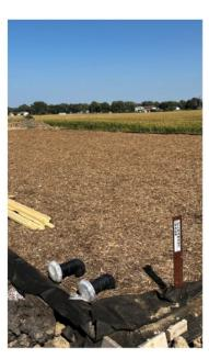
The first photo is in Beresford where the hole has been dug, the HDPE Liner has been installed and the piping is in place. The next step is the rock. In the second photo, the SAGR rock is being installed into the lined ponds. The last photo is from Worthing. This is the finished project with 1.5' of mulch over top for insulation.
